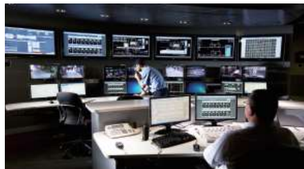
Command and control center
